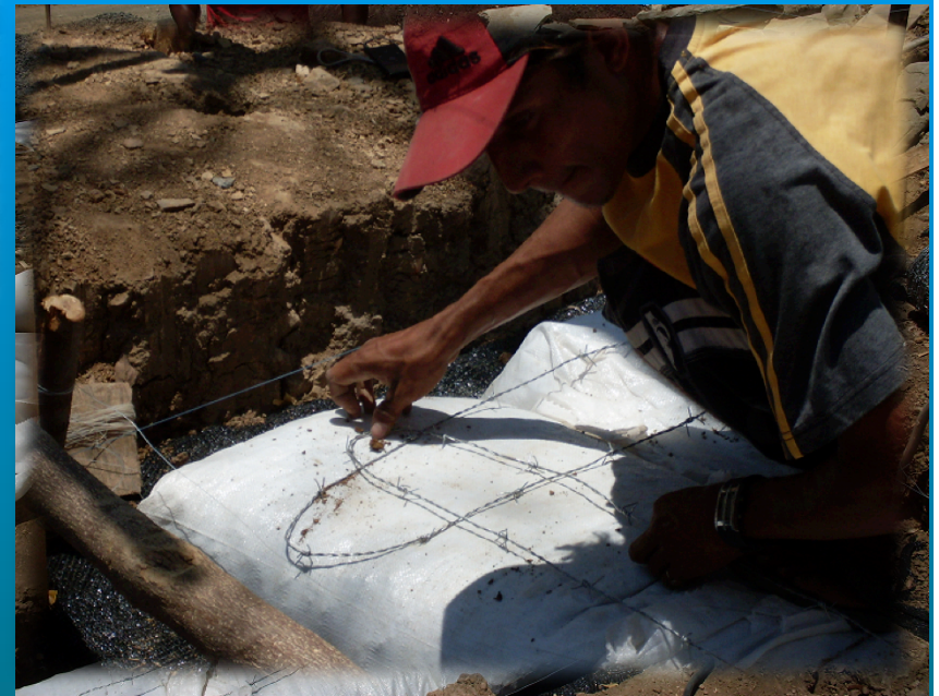
Reinforcing lateral strength between bags
